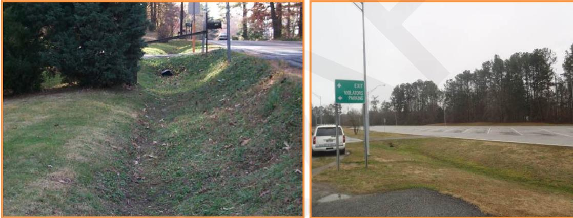
Figure 5.2-1 Two Examples of a Roadside Grass Channel
