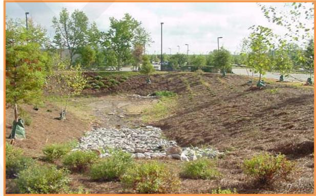
**Figure 5.6-1** Dry Detention Basin with Low-Flow Channel (left) and Dry Detention Basin with Landscaping (right)
