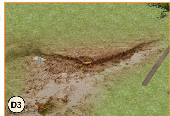
low-flow channel is present. Ensure that the entire bottom of the basin slopes toward the channel.
